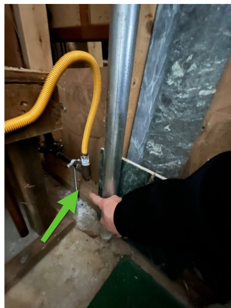
Missing sediment trap.
